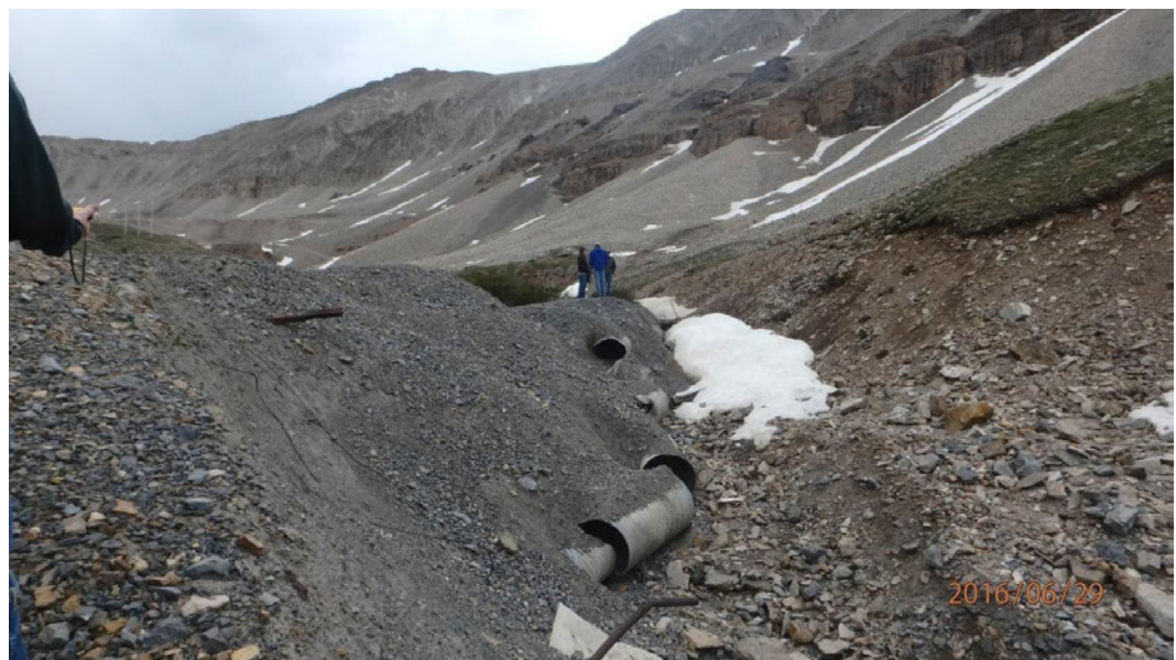
Figure 7. South Channel depicting severe incision and downcutting that has occurred over the years. This sedimentation and erosion will continue to occur and create an unstable environment until this project is completed.
