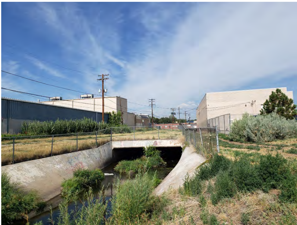
Current state of the concrete channel and undersized culvert at Weir Gulch.
