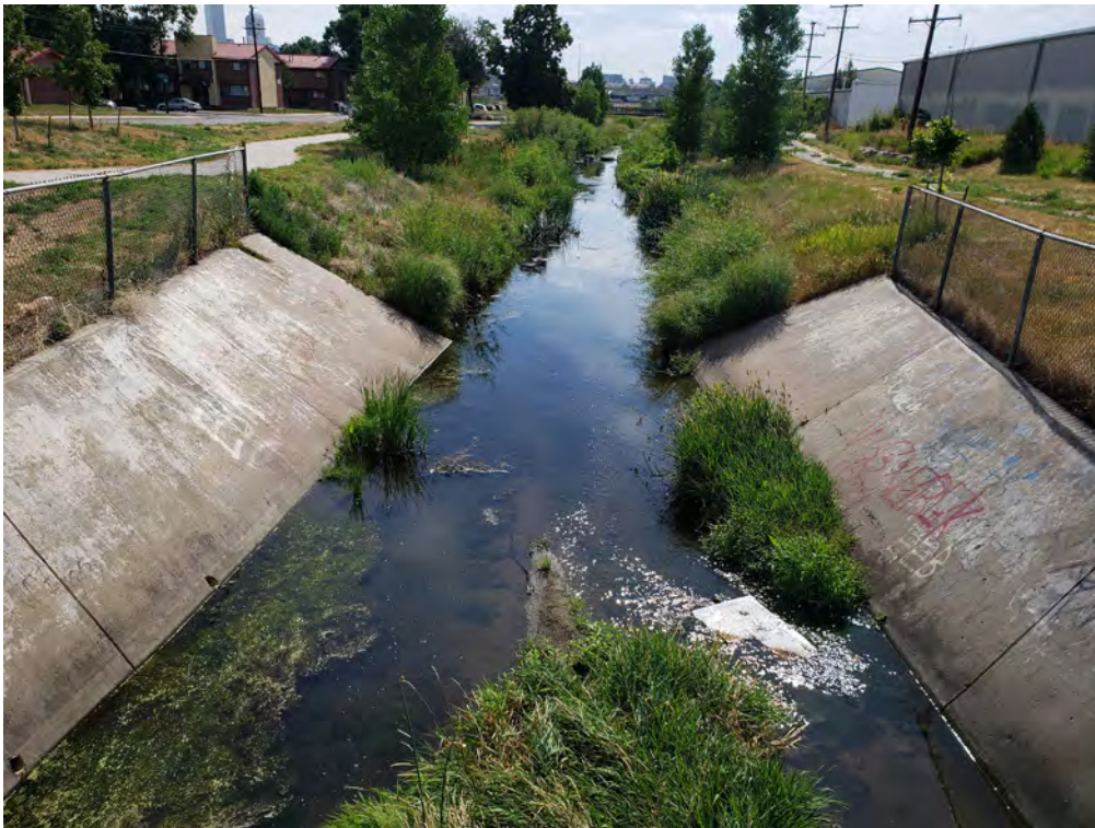
Looking downstream along the existing concrete channel at Weir Gulch. The upcoming project will convert this channel into a more naturalized waterway, improving flood management, enhancing ecological habitats, and integrating recreational paths for community use.
