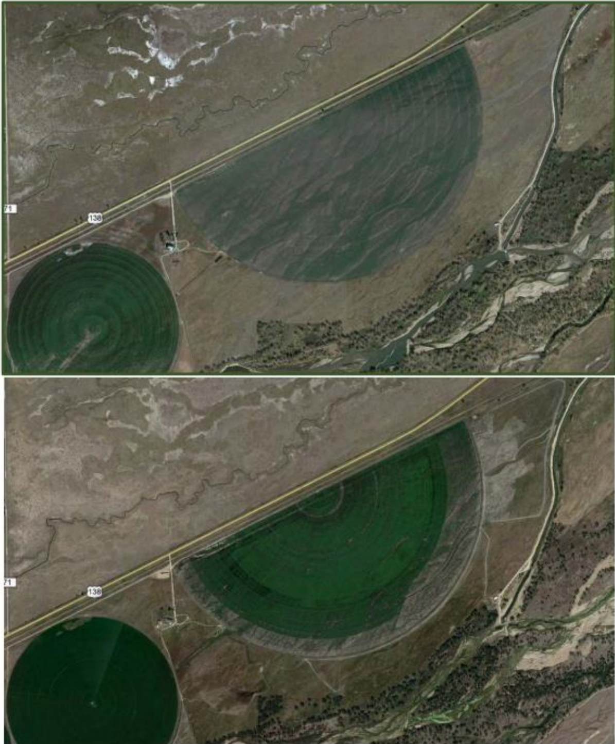
Photo: Set of aerial images of the LaFleur Wetlands project site from pre-project delivery (October 2015 - top) and post-project (September 2020 - bottom) showing installation of wetland infrastructure.
